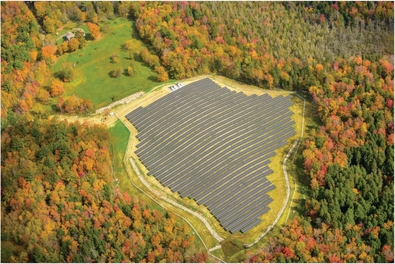
Eversource Massachusetts Solar Facility in Hinsdale, MA (2.75 MW)
